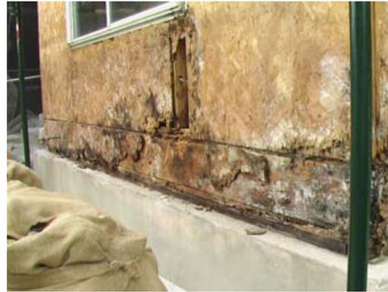
stone wainscot on his home in the Alaskan Bush, we stacked 15 sheets or so of mixed plywood against a tree outside. After only a month of being exposed to the Alaskan humidity, the O.S.B. plywood in the stack was covered with mold while the CDX plywood looked like new.
